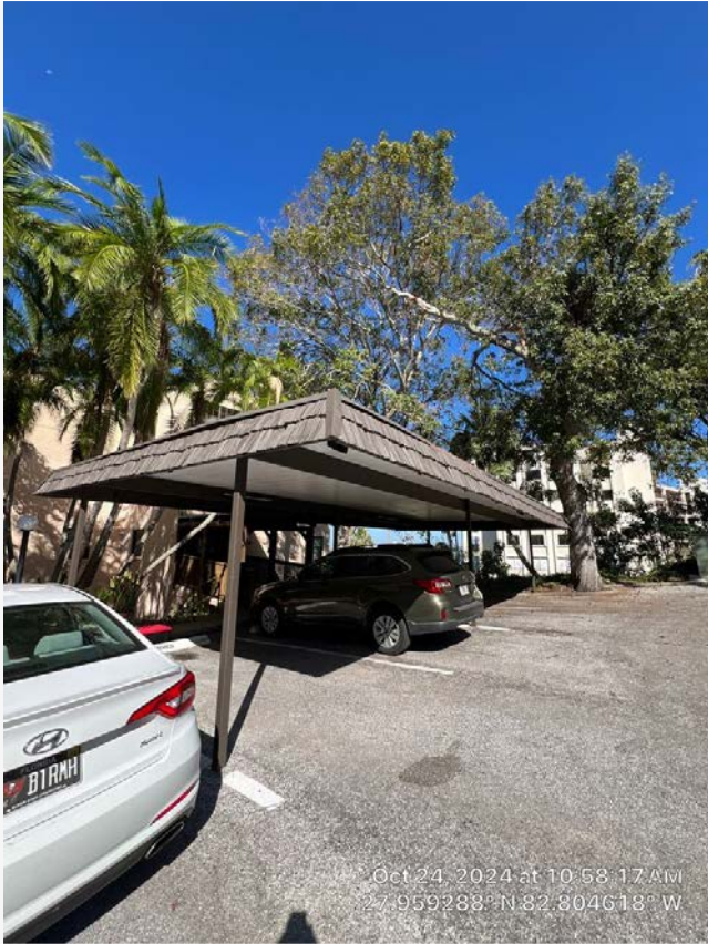
Carport in front of east elevation for 9 Turner units.
