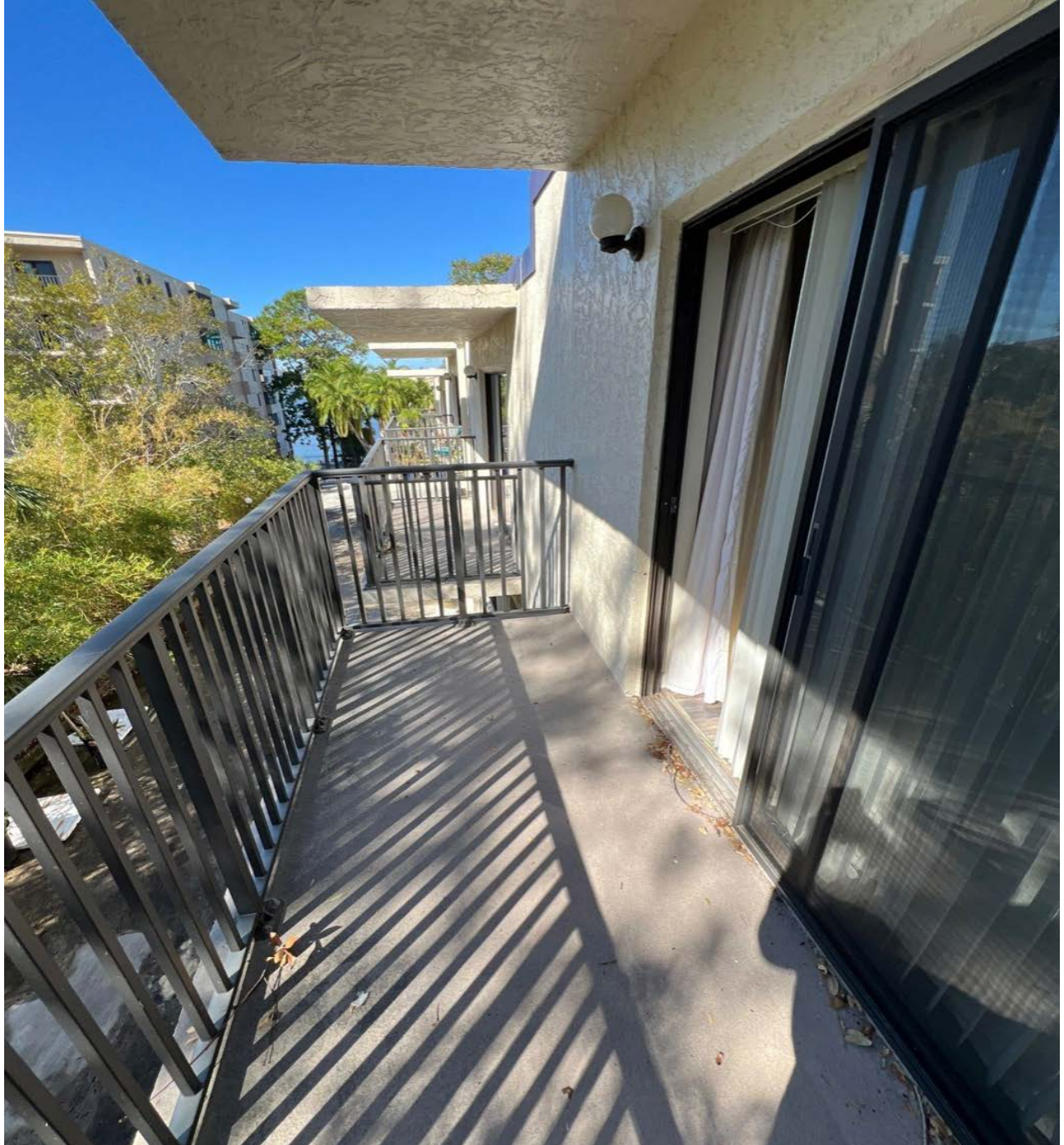
15 Turner St. - Unit 2 South Balcony
