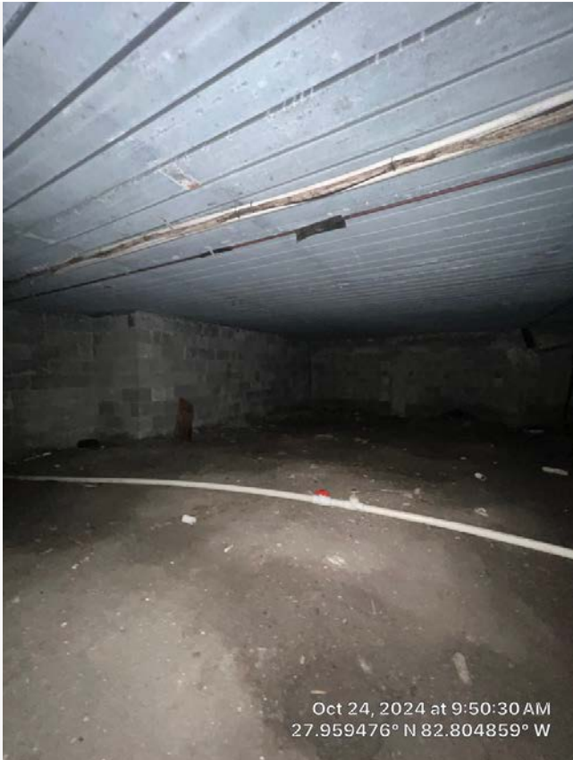
Crawl space under building. No issues observed.
