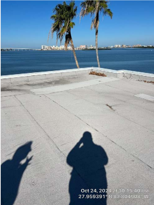
Roof view looking to the northwest.
