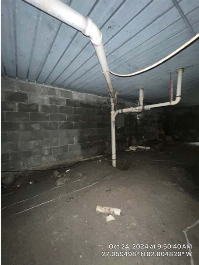
Crawl space under building. No issues observed.
