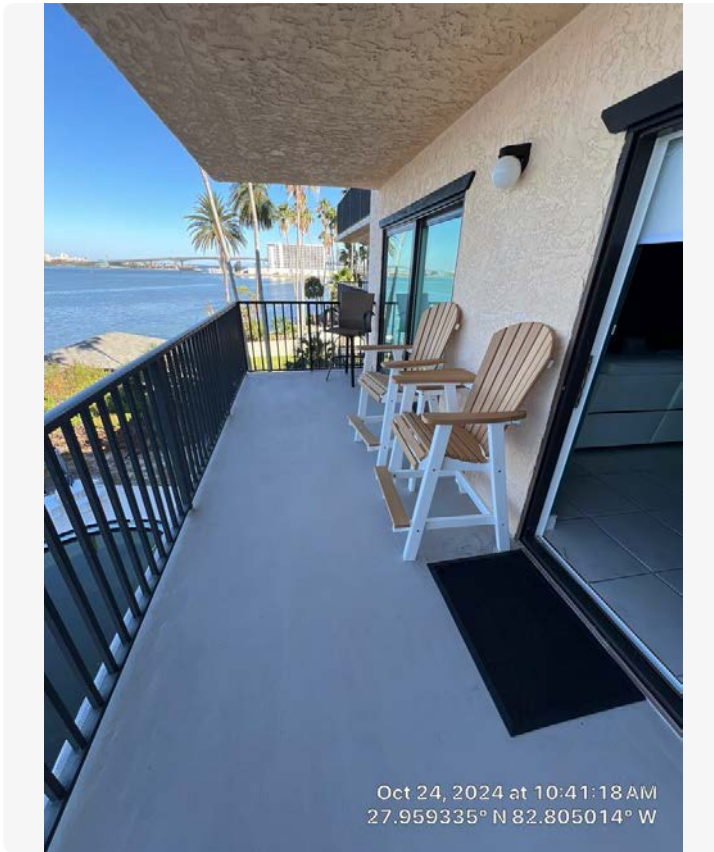
North facing view balcony of Unit 12.
