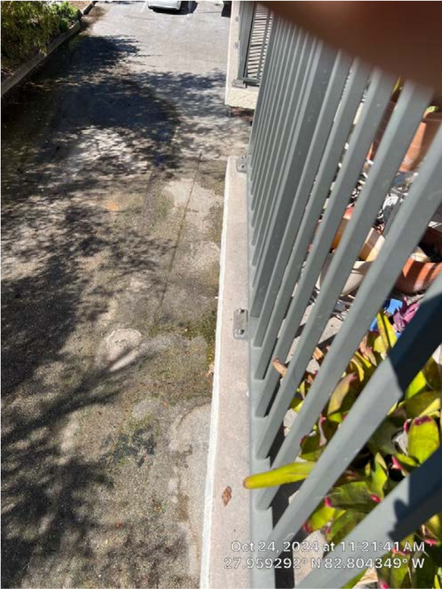
View to the west of south balcony slab edge Unit 4.
