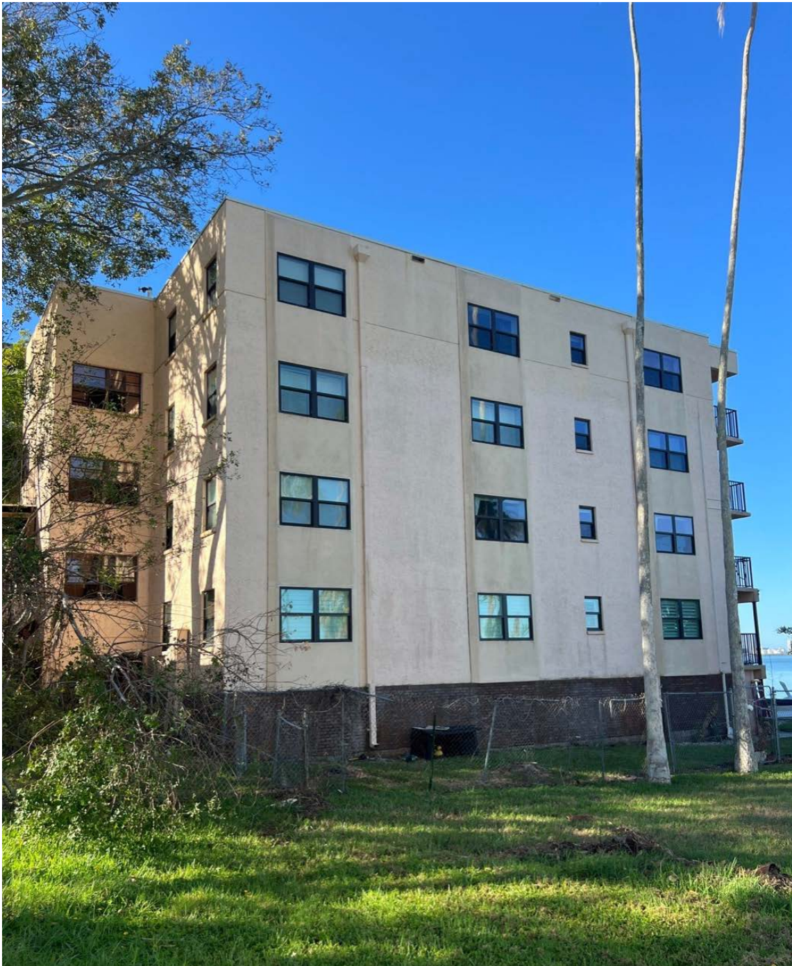
9 Turner St. - Side (North) Elevation
