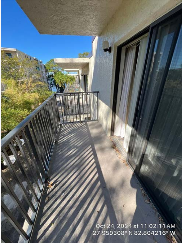
Unit 2 south balcony.
