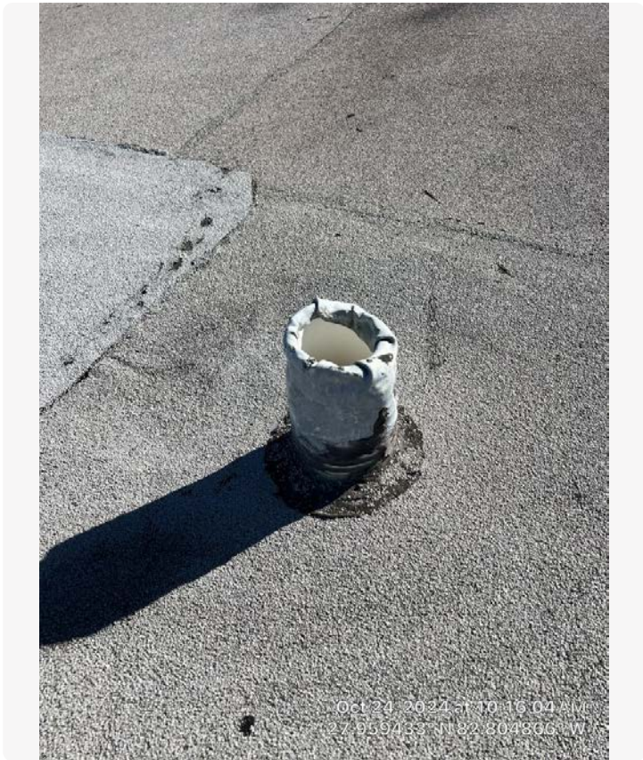
Vents appear to be in good condition and free of debris.
