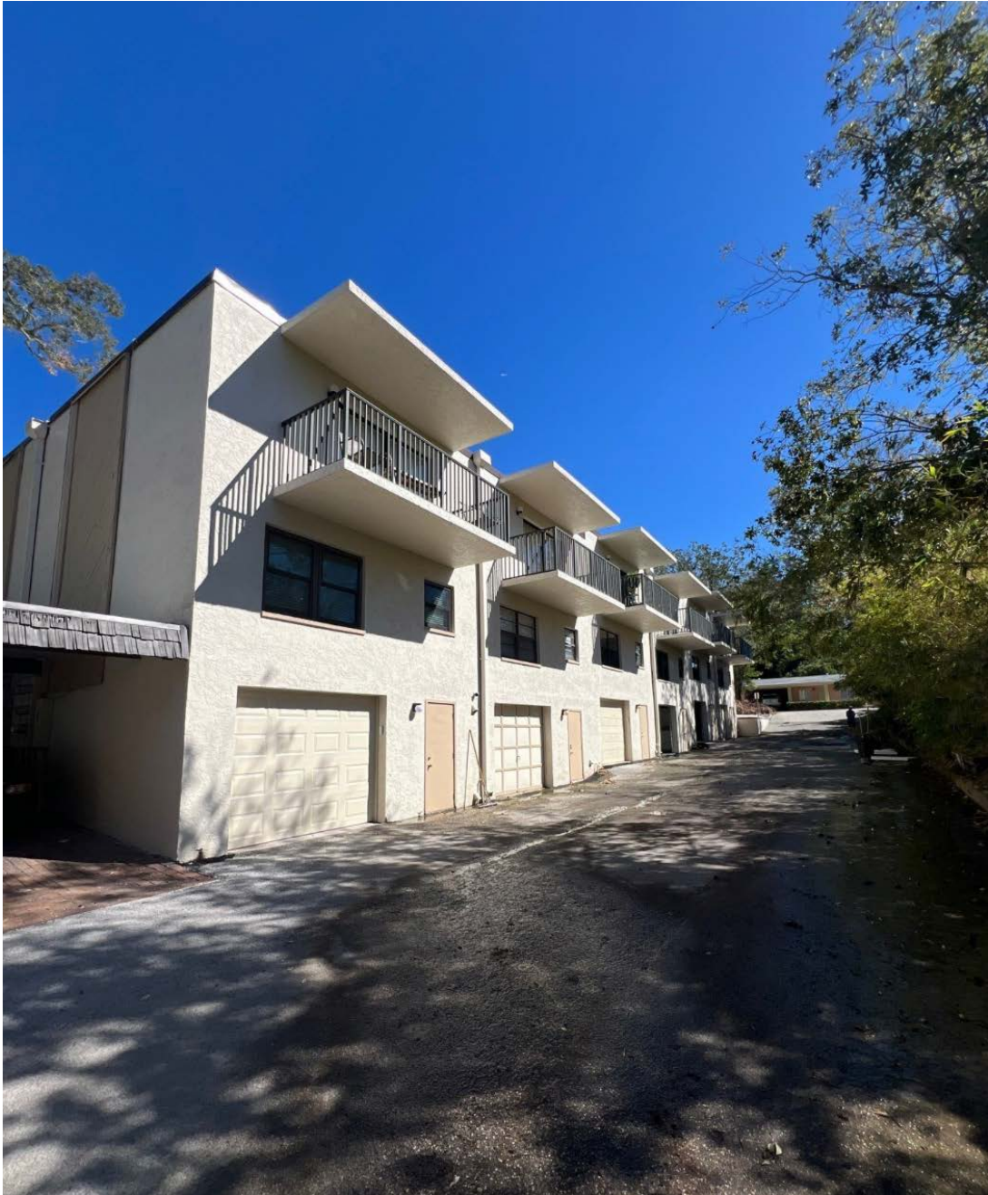
15 Turner St. – Rear (South) Elevation
