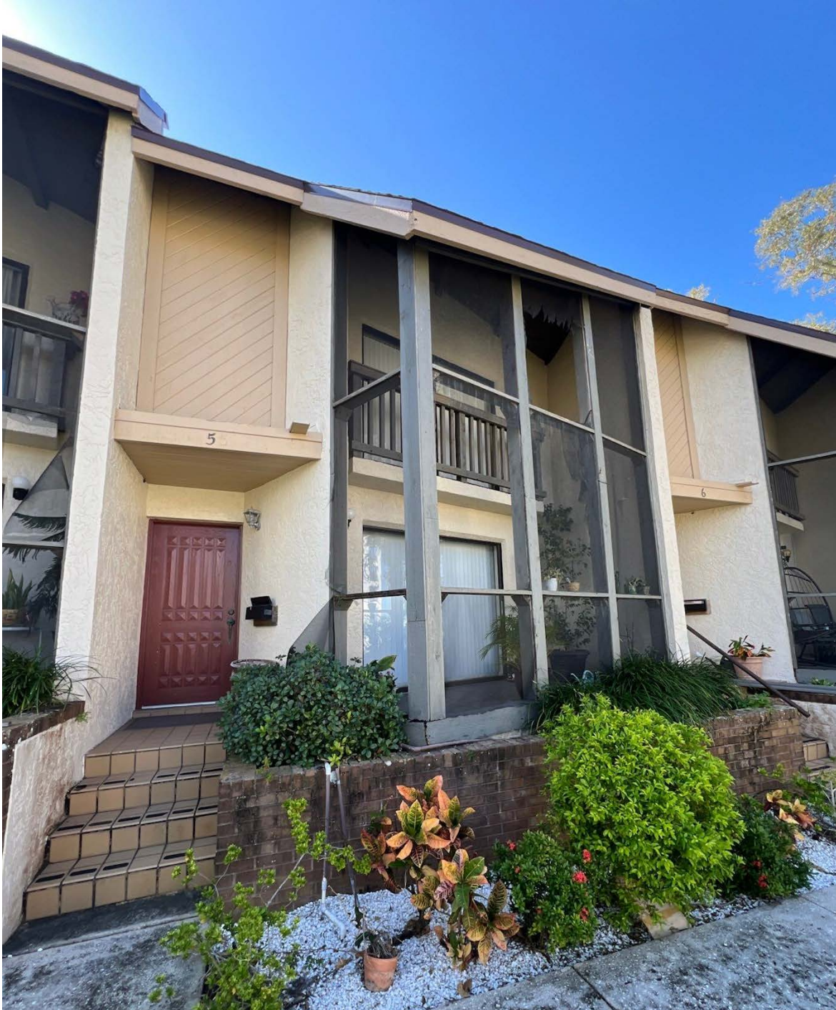
15 Turner St. - Unit 5 Porch Enclosure (North Elevation)
