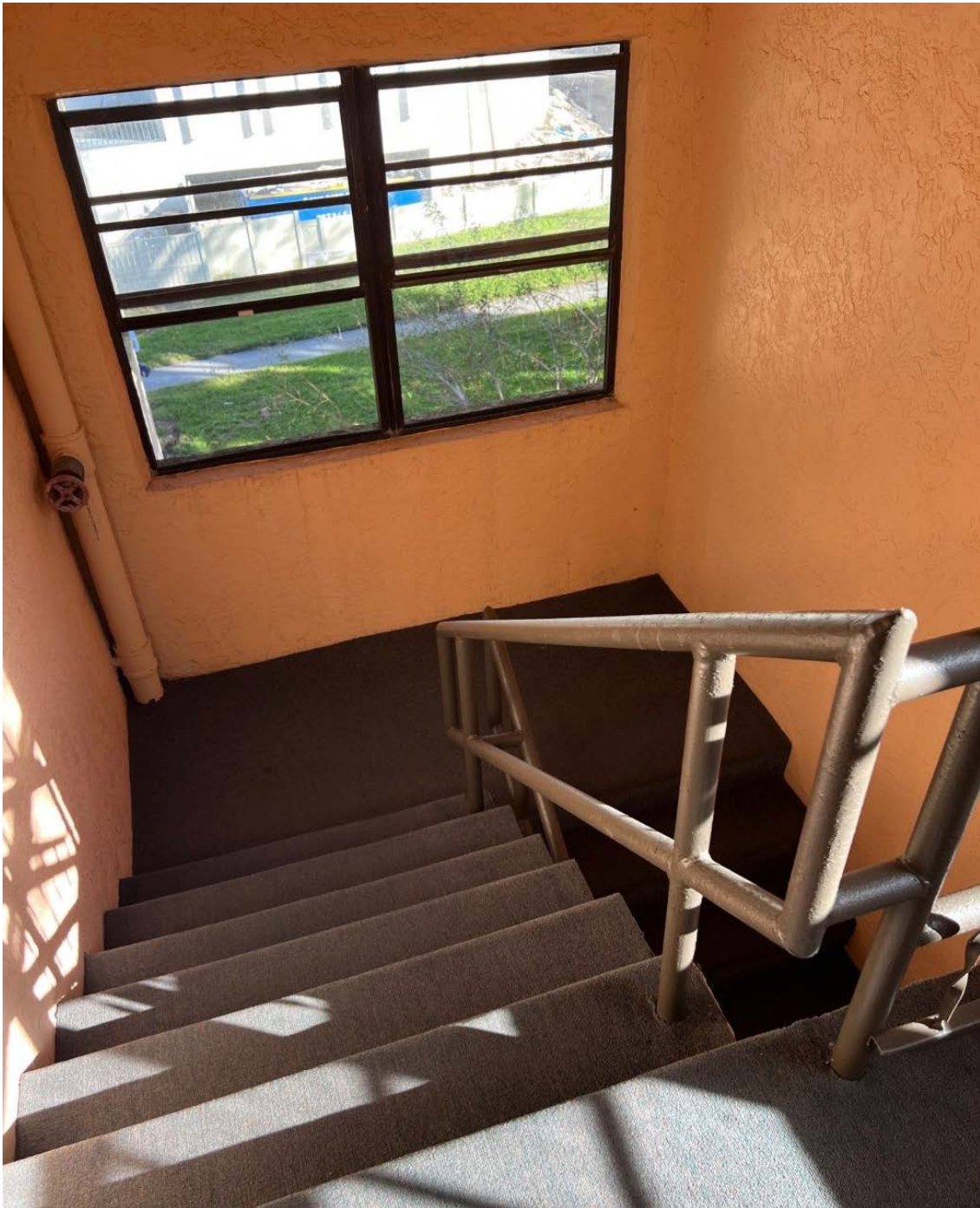
9 Turner St. - Front Stairwell
