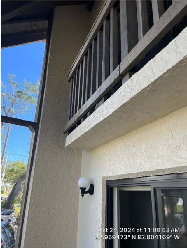
Unit 1 north balcony slab edge.
