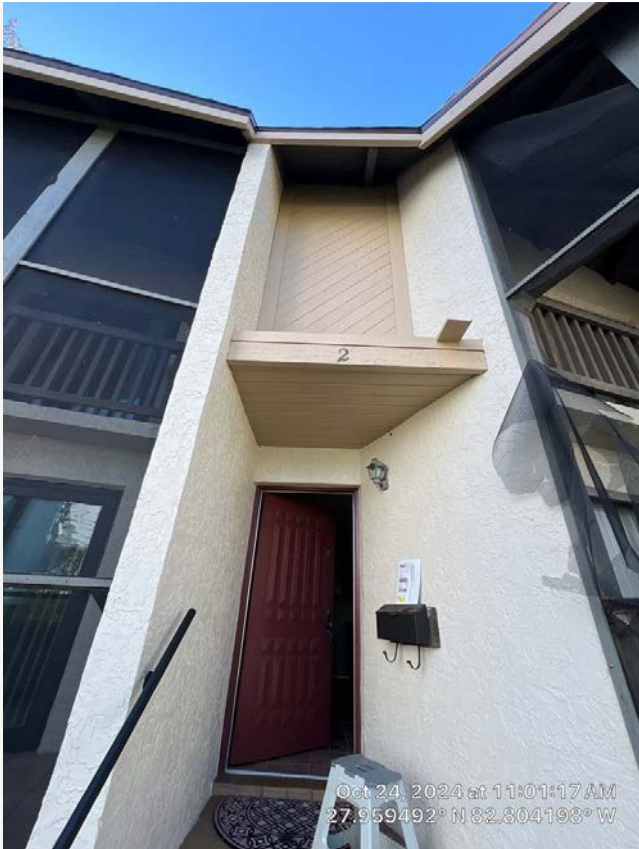
Unit 2 front elevation (north).
