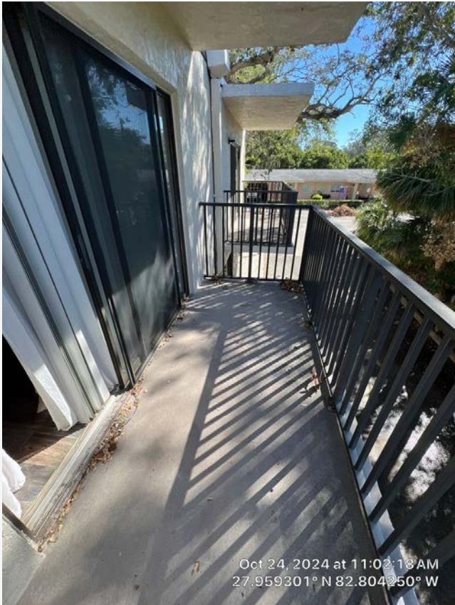
Unit 2 south balcony alternate view.
