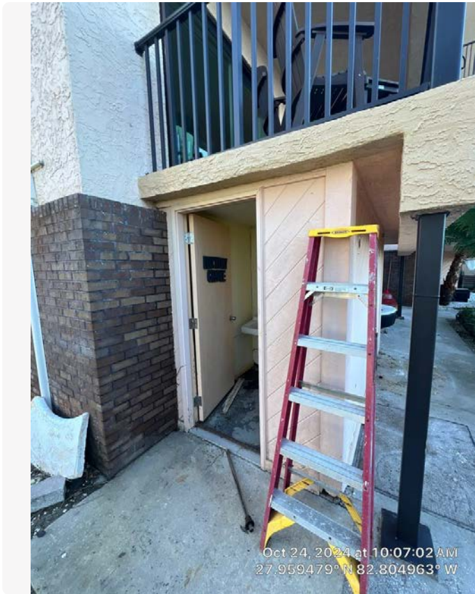
Northwest elevation mens room.
