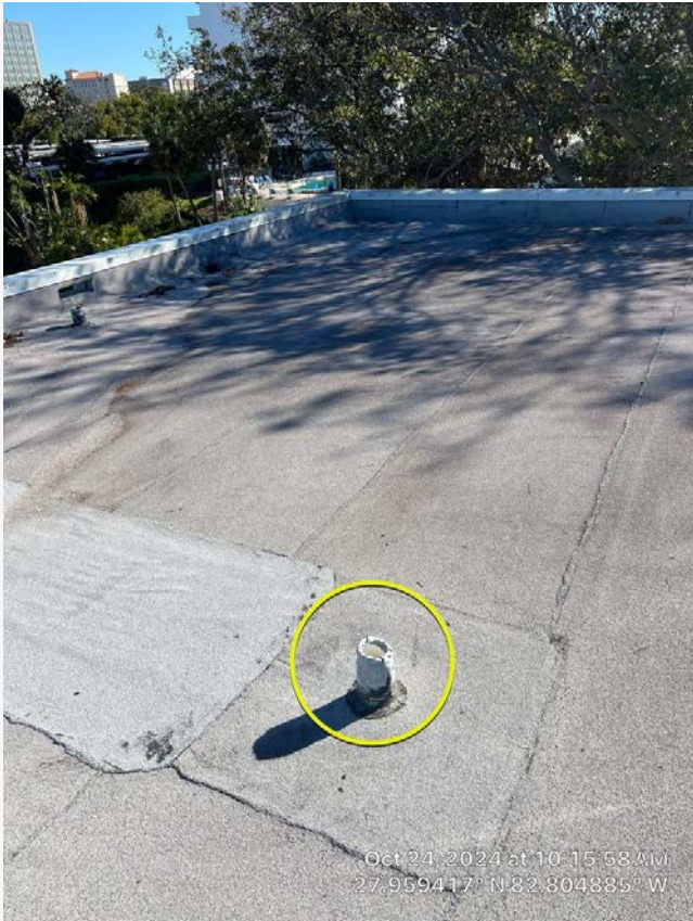
Vents appear to be in good condition and free of debris.
