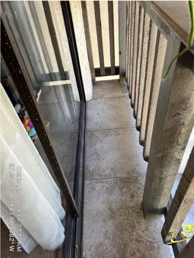
North balcony Unit 4.
