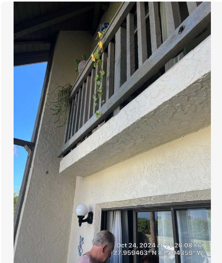
North balcony slab edge Unit 4.
