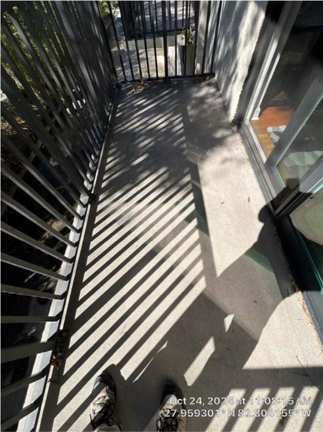
Unit 1 balcony general conditions.
