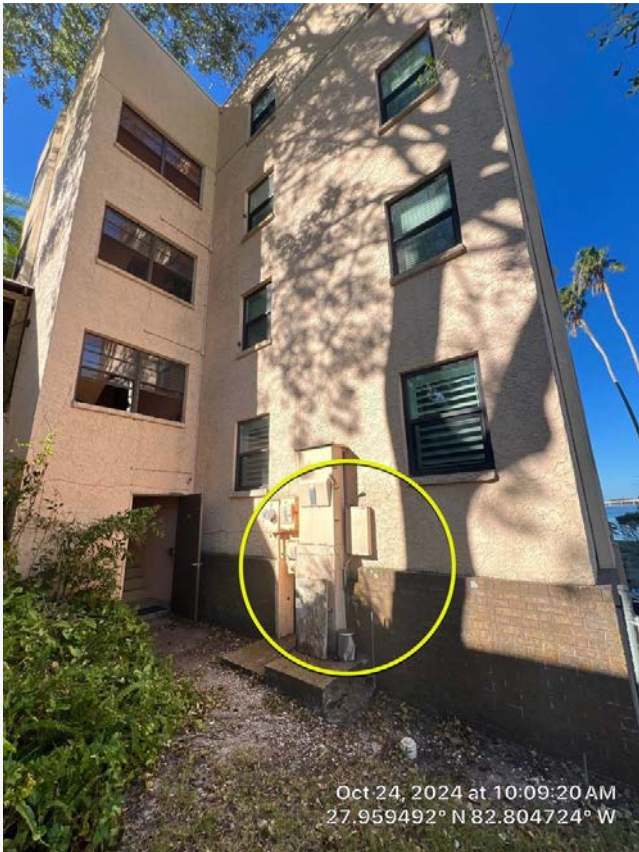
Front east elevation. Cracking in stucco observed. This crack should be repaired to prevent moisture-induced deterioration of the stucco.
