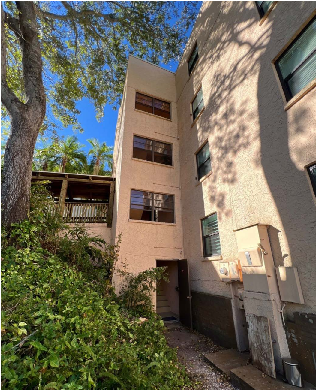
9 Turner St. – Front (East) Elevation - Stairwell
