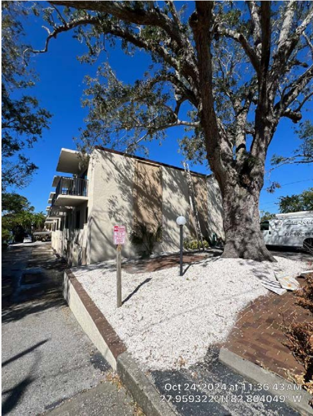
Side (east) elevation.
