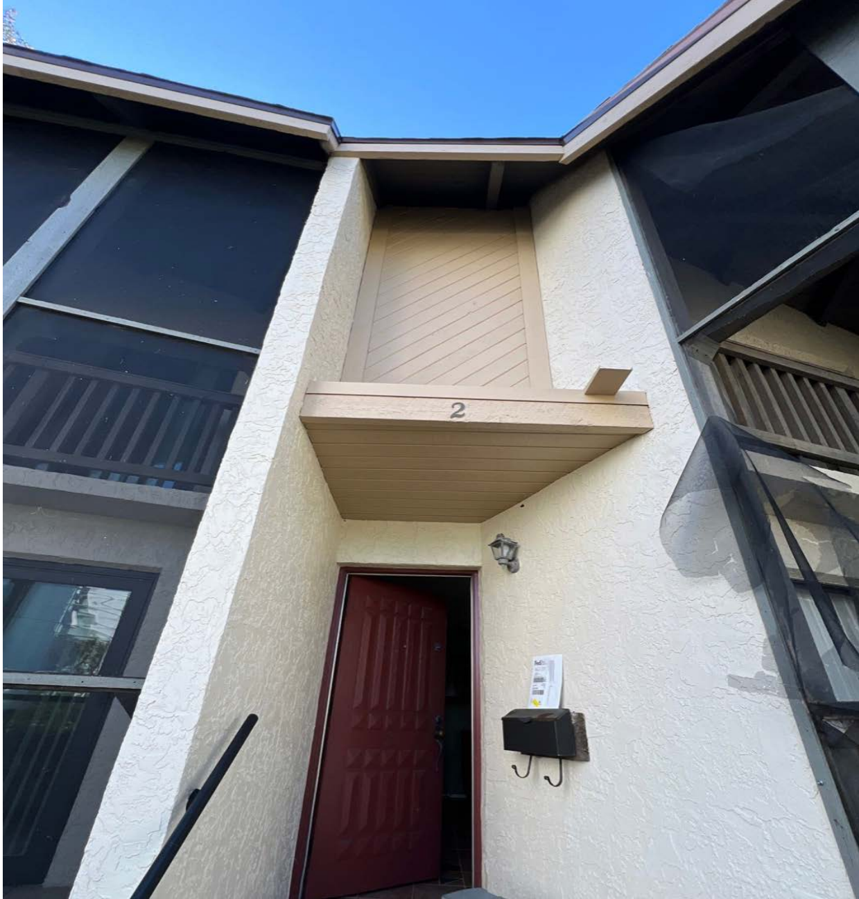
15 Turner St. - Unit 2 Front (North) Elevation
