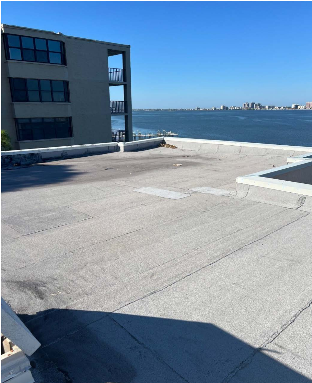
9 Turner St. – Roof View Looking Southwest
