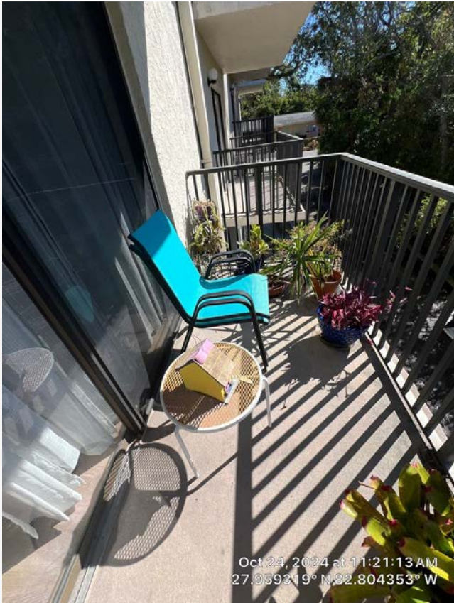
South balcony of Unit 4.
