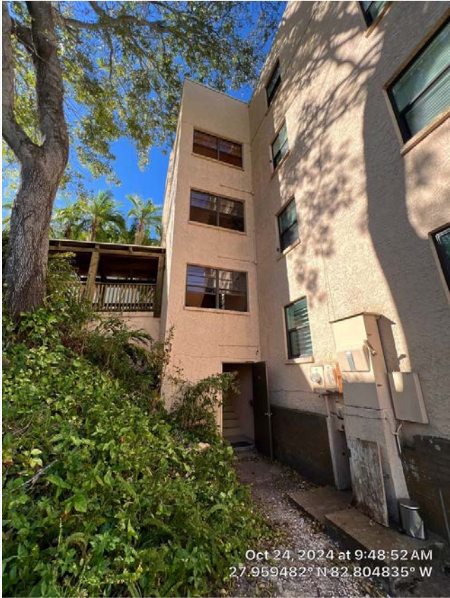
Front stairwell east elevation.
