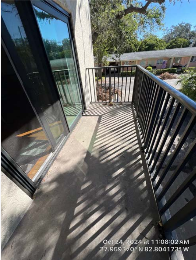
Unit 1 south balcony.
