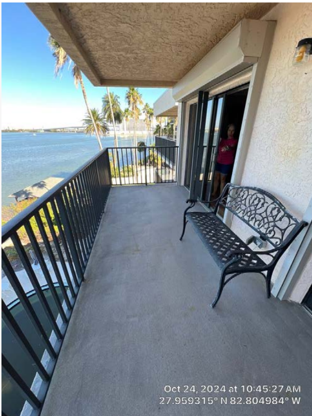
Unit 14 alternate balcony view.
